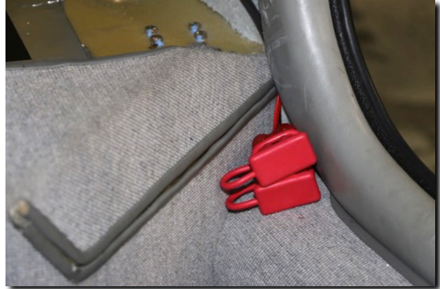
SB50 charger plugs with protective covers.
